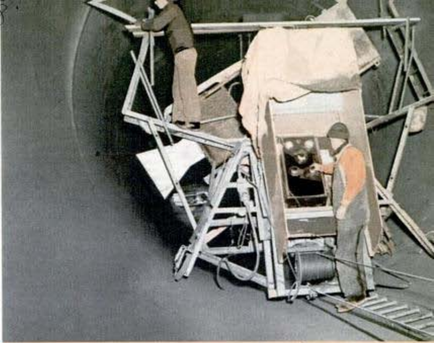
↑ Portable X-ray machine rolls into the 18-foot penstock to examine its welded joints for any hidden flaws
